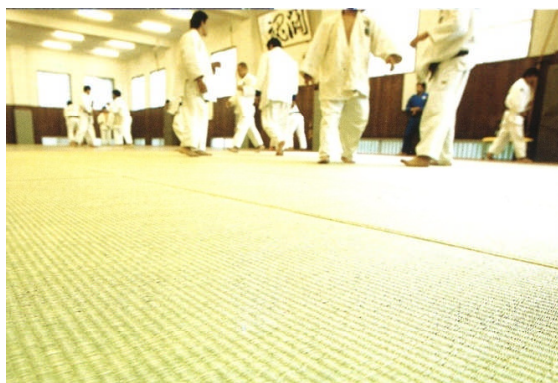
Fig32: Judo hall equipped with tatami mat covered with Shichitoui sheet
